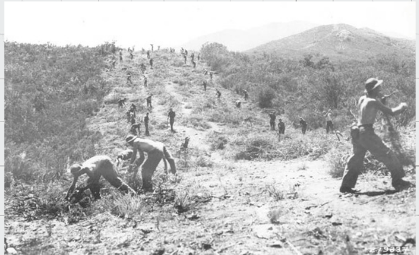
CCC staff constructing a fire break in the San Bernardino National Forest in June of 1933. Photo by the Forest History Society.
